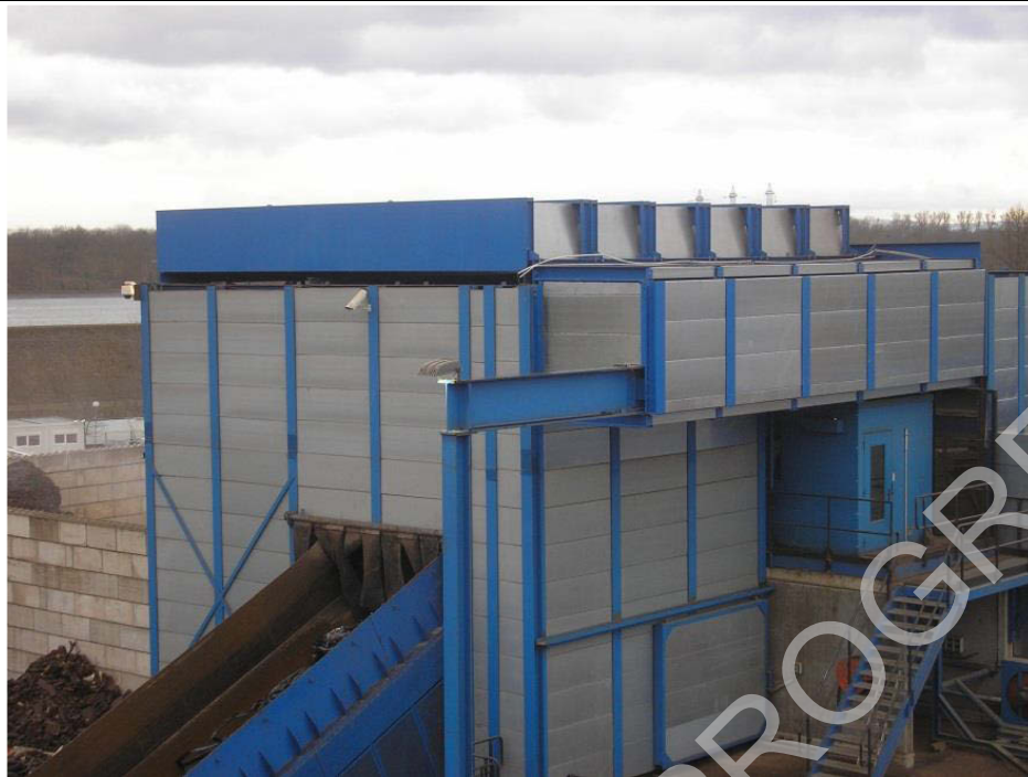
Figure 3.24: Splitter silencers at the roof of a shredding plant
