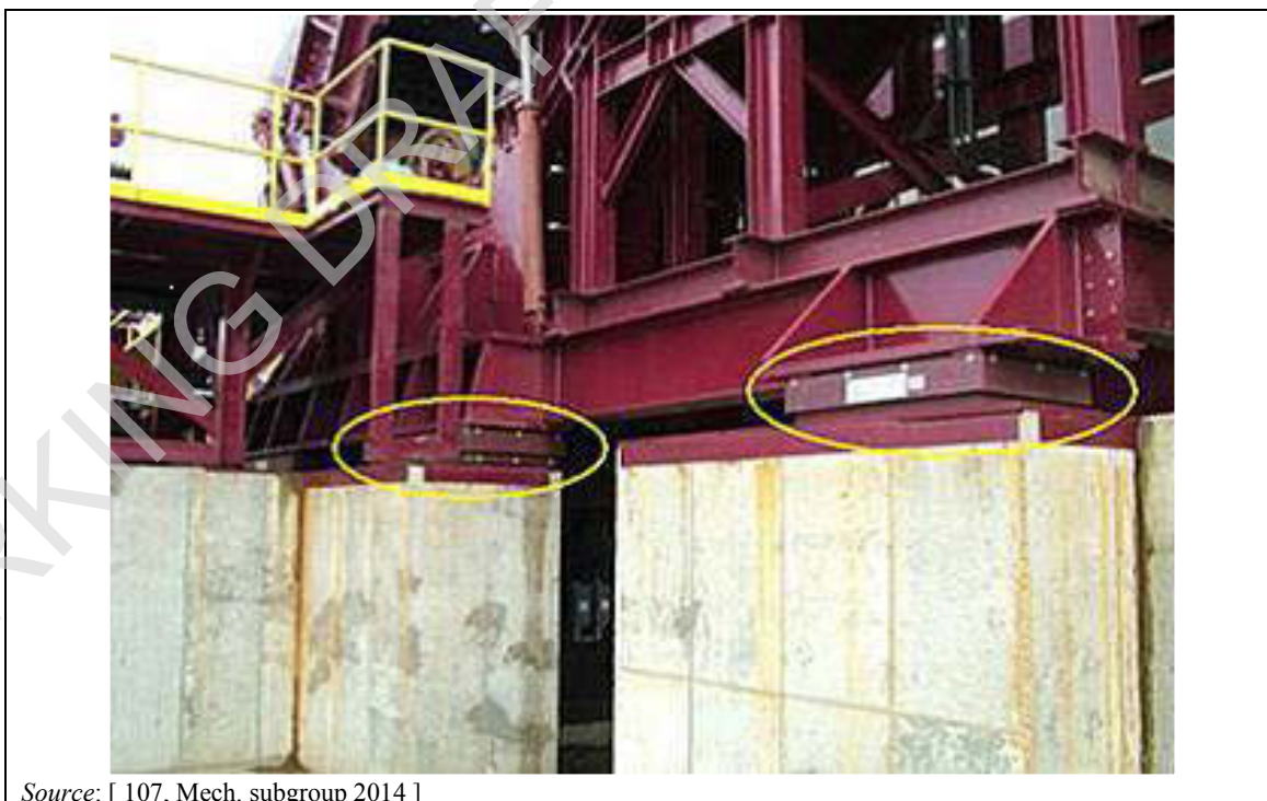
Figure 3.22: Isolation elements (circled) for vibration reduction
