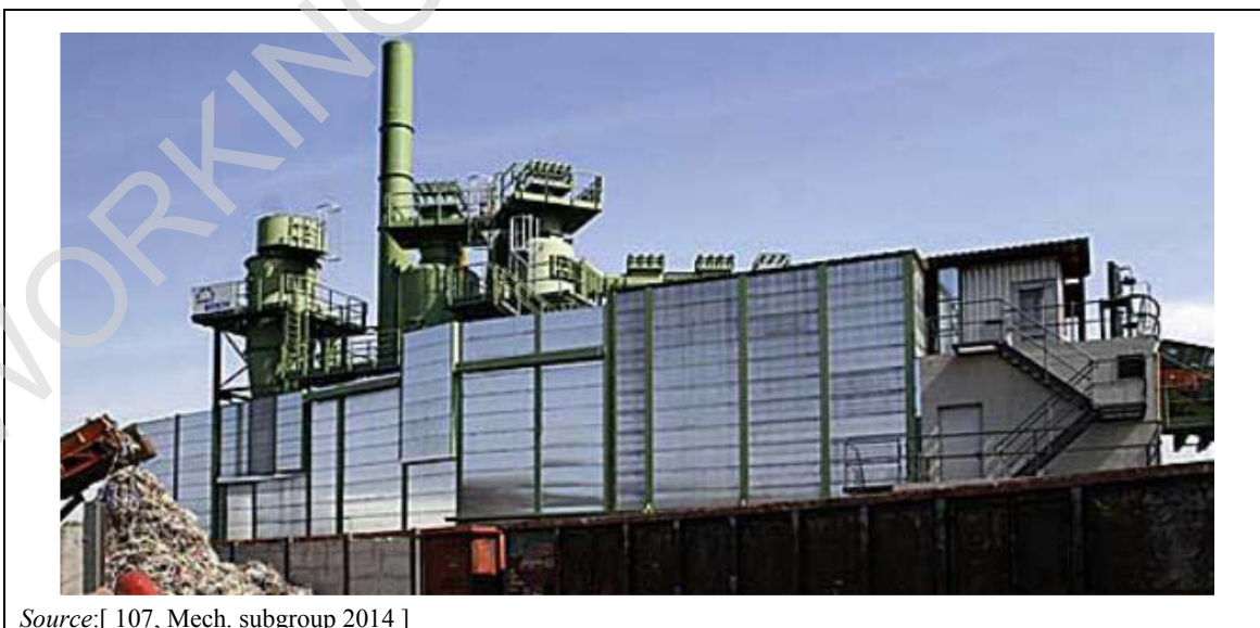
Figure 3.23: Protective screening at the Schrott-Bosch GmbH shredder, Germany
